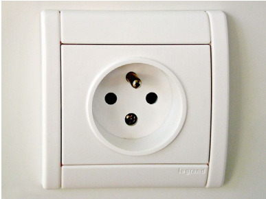
International Commission on the Rules for the Approval of Electrical Equipment (IECEE) CEE 7/5
